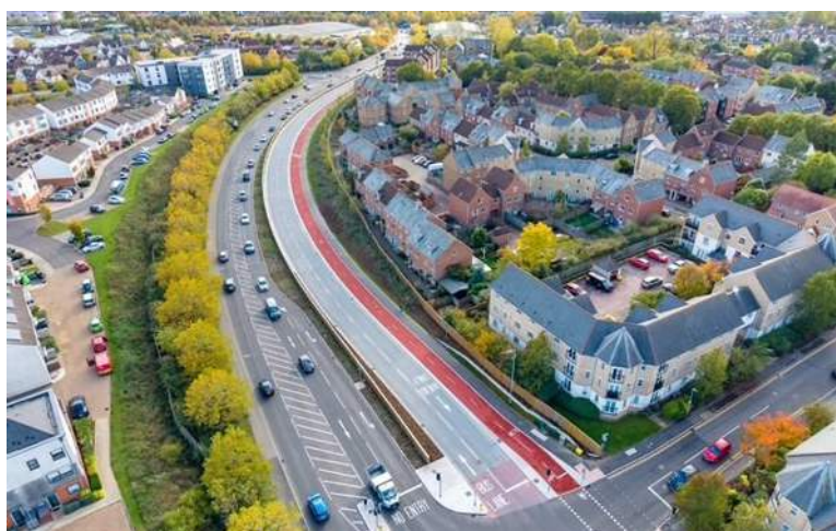
Figure G.1: Integrated RTS, cycling and walking infrastructure completed in 2025
